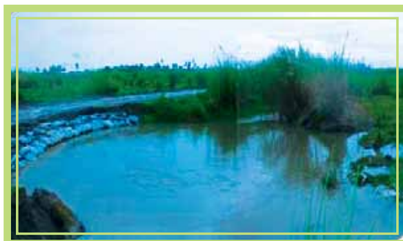
REGION 12 - Lambayong RIS, Sultan Kudarat Damaged protection dike affecting 13 barangays of about 3,100 ha. isolated area in the system since wet season of CY 2008.
