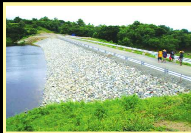
San Angel SRIP, Rosales, Pangasinan. Construction of a zoned earth fill dam 13.50 meters high, with a crest length of 120 meters, and reservoir storage capacity of 0.289 mcm to irrigate 161 has.
