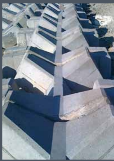
Tetrapod concrete blocks weighing about 2 tons are laid as strong slope protection of dikes. (East Area of Sendai).
