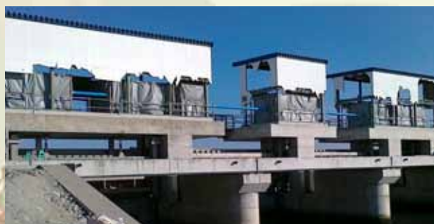
While the reinforced concrete tidal drain gate structure (operating platform and bridge) withstood the tidal onslaught, the electro-mechanical equipment and its enclosure did not (East Area of Sendai).
