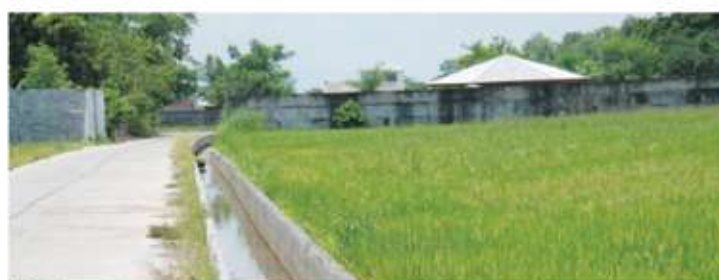
Lining of farm ditches / canal is one of the main projects of PIA as model IV IA
