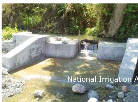
Gabion spurdiike, spill way and CHB lined canal of Kamantilis CIS
