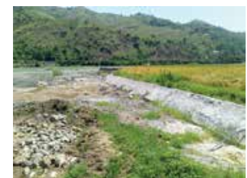
Gabion spurdiike, spill way and CHB lined canal of Kamantilis CIS
